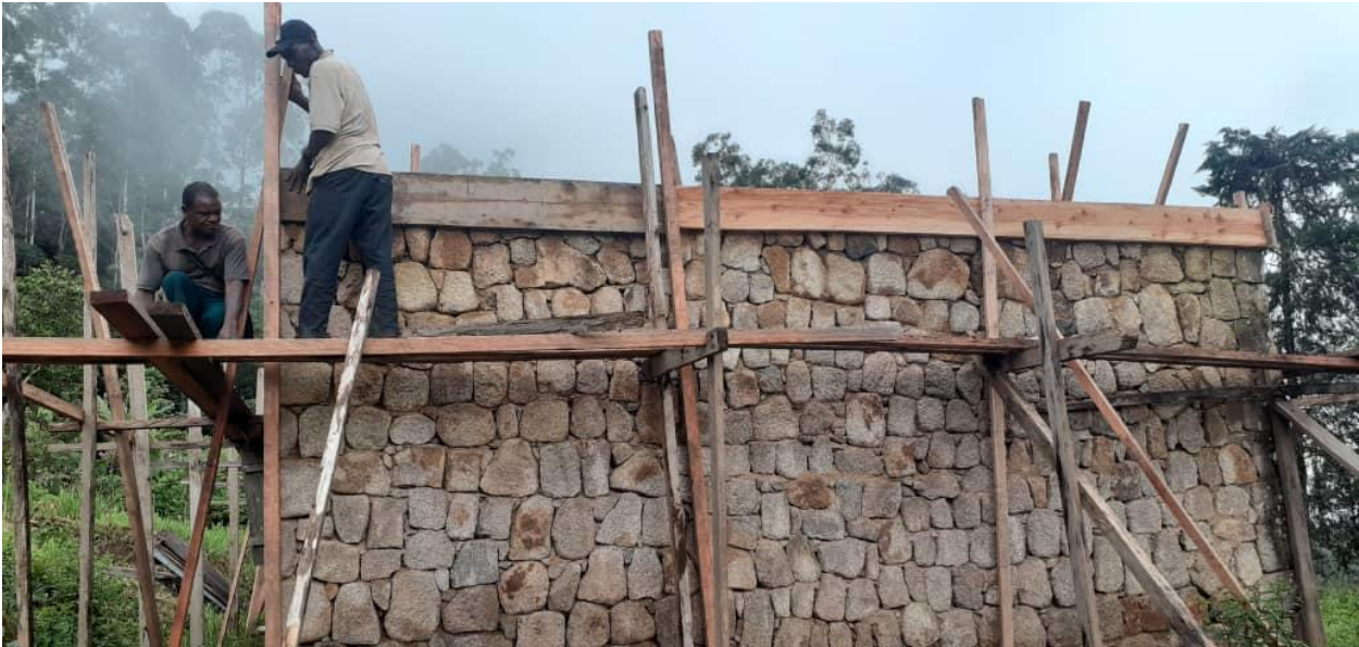
Construction of Roof reinforced concrete beam
