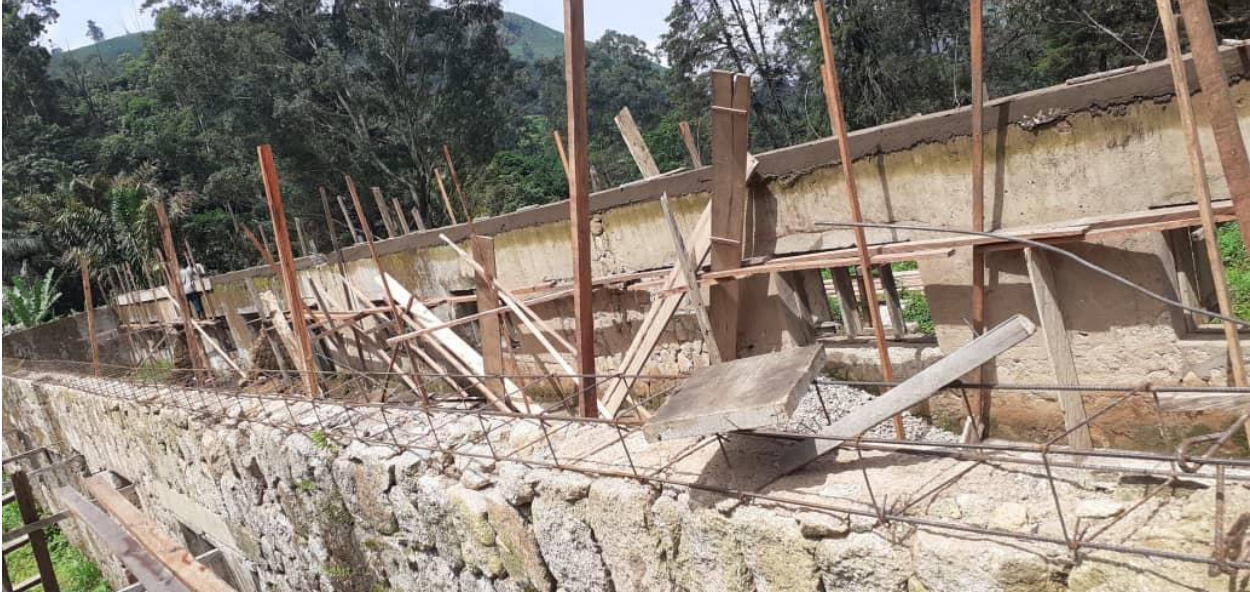
Construction of Roof reinforced concrete beam
